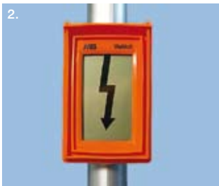
1. Pilot installation on ENION S.A. distribution station, Krakow, Poland | 2. Status – voltage on | 3. Status – voltage off.
